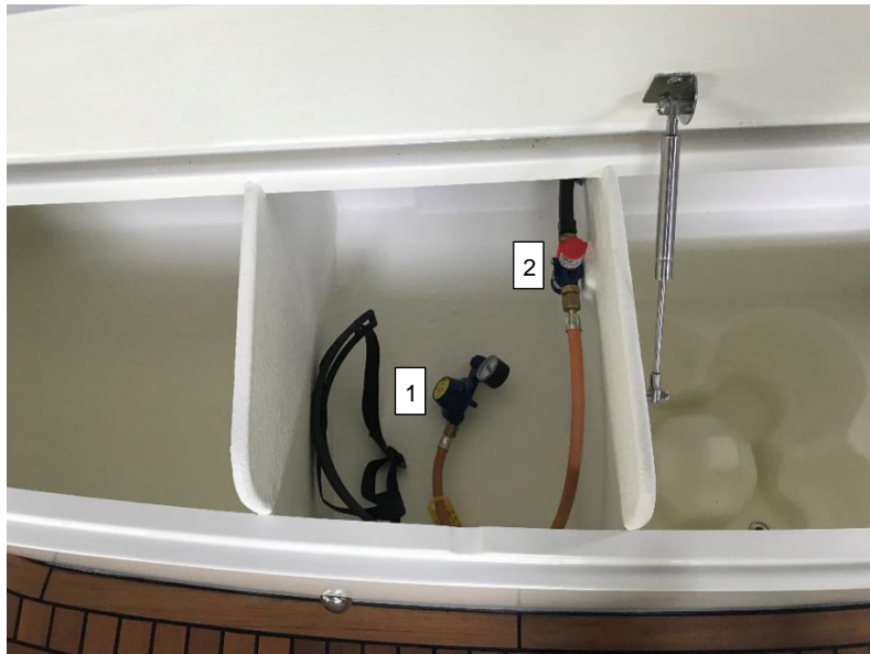
Picture 57: Gas bottle - the pressure reduction valve (1), the test button (2)
