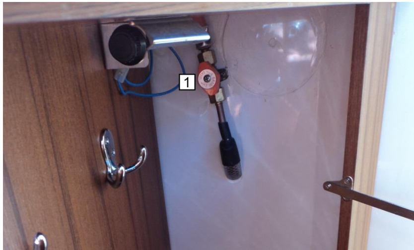
Picture 8: Gas closing valve for cooker and oven (1) is inside of the trash closet in the pantry
