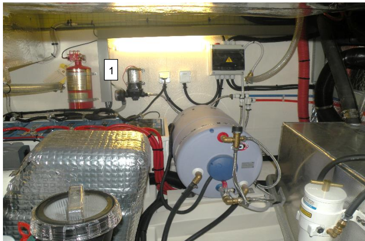
Picture 24: Fresh water pump and filter in the engine room (1)
